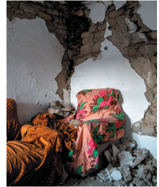
Their house was highly dangerous to enter and had to be condemned.
